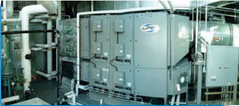
Hearst Tower installation
